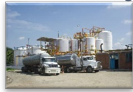
Bulk Gas Storage
