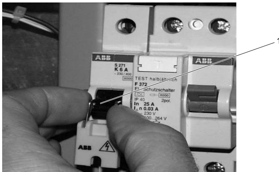
Fig. 28: Remove the safety clip of the Pre-fusing
